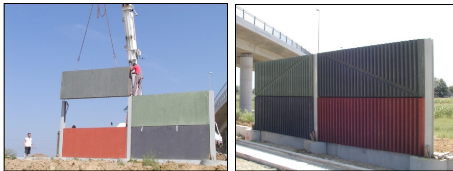
Figure 5 Installation of test section of RUCONBAR panels
